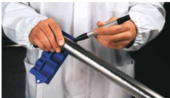
Figure 28 - Marking the insertion depth
