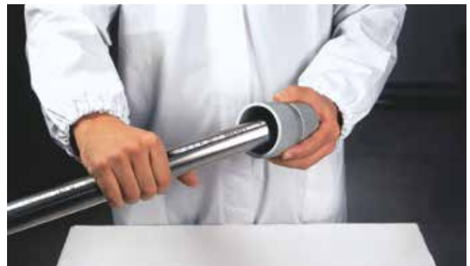
Figure 26 – Deburring the pipe
