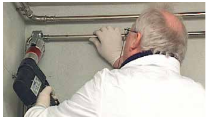
Figure 32 – Making the press connection
