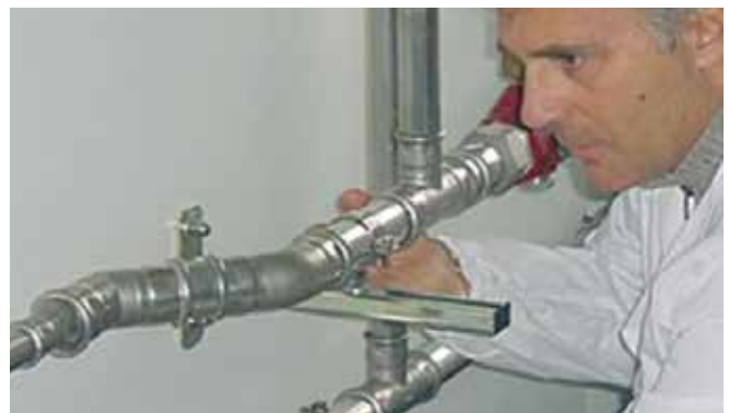
Figure 33 – Checking the press connection
